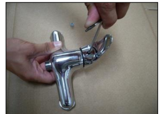
2 - loosen the screw of the handle
